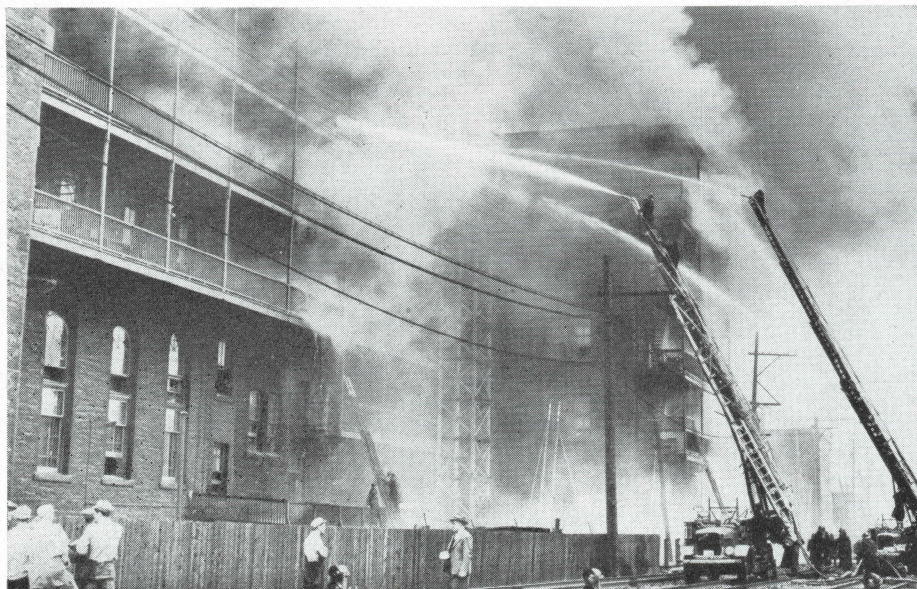
HOSPICE HOLOCAUST — Montreal firemen battle in vain to save the fiercely burning St. Cunegonde Catholic Home for the Aged, Blind and Orphans on June 15. The outbreak occurred during welding operations. Flames swept up the elevator shaft, quickly turning the six-story structure into a raging inferno. Of the 300 persons housed in the building, 37 lost their lives and many were injured
