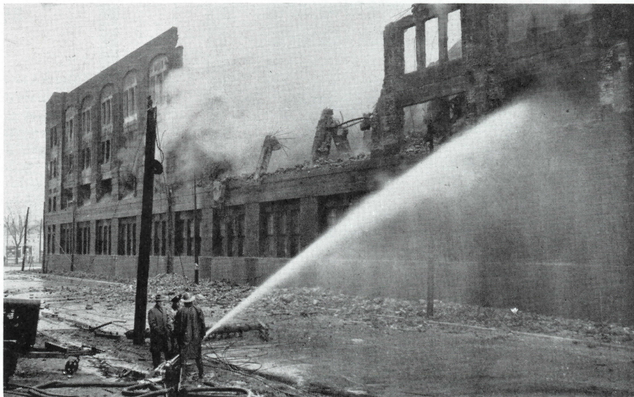
DELAYED ALARM AIDED DISASTER —Destruction of this four-story fire-resistant building in North Kansas City on March 15, 1950, followed delay in notifying the fire department while employees futilely tried to extinguish the flames. The loss, including damage to an exposed building, was $3,195,000
