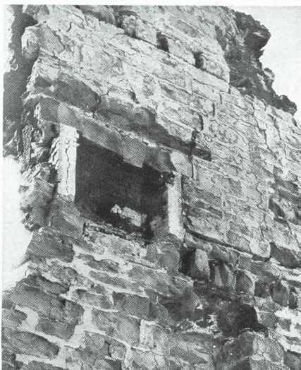
DEFECT CAUSED DISASTER —Nine Kenyon College (Ohio) students lost their lives on February 27, 1949, when a defect in this chimney allowed smoke and fire to enter floor and wall spaces of 122-year-old dormitory. Eventually a hole was burned through the first-floor ceiling and the blaze consumed the building in a matter of minutes
