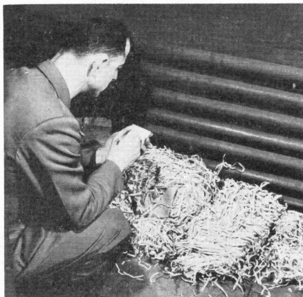
DANGER POINT — Paper packing material placed too close to heating pipes constitutes a real danger. Fire safety inspector will report condition to plant "fire chief" for prompt correction
