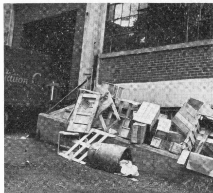
COULD BE COSTLY — Careless disposal of boxes, oil drums, loose paper and other combustible materials is hazardous. All such refuse should be deposited in a safe place away from buildings
