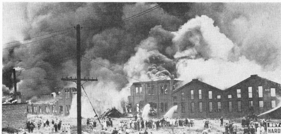
OIL-SOAKED FLOORS FED FLAMES which swept this Jersey City steel plant following delayed alarm. One man was killed and six others were injured
