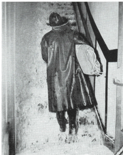
MAN-MADE WATERFALL — Typical salvage operation shows fireman mounting stairway down which water has been diverted to prevent a ceiling collapse. Canvas blanket under his arm will be used to protect merchandise from damage
