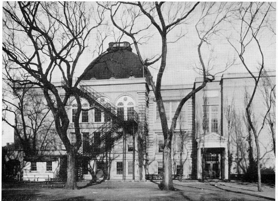
PUPILS PROTECTED —Memminger School, Charleston, S. C., where Aero System gave timely warning when boiler safety device failed. This is one of the eleven Charleston schools in which Aero has been installed to protect the lives of pupils and taxpayers' property
