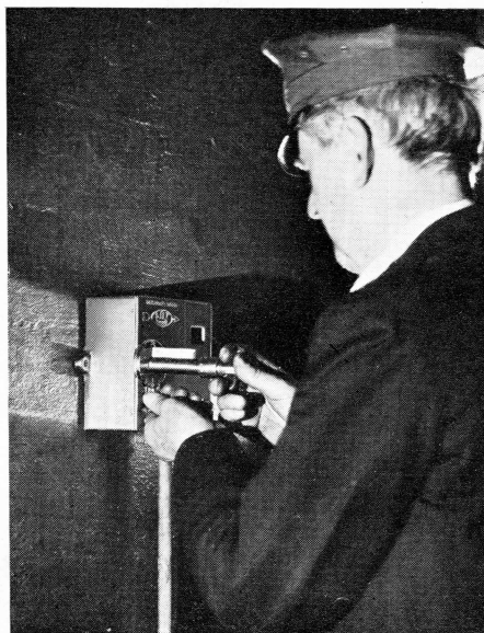
"A FRIEND IN NEED" is the A.D.T. Watchman Supervisory Patrol Box, through which the watchman signals the Central Station at predetermined intervals. If a signal becomes overdue, A.D.T. Guards immediately dispatched to investigate
