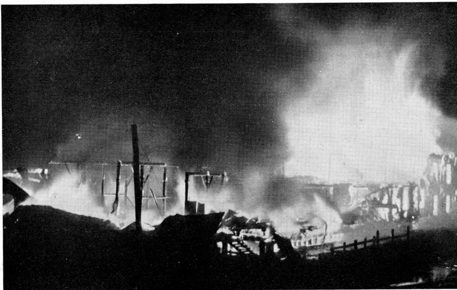
GENERAL ALARM FIRE destroyed this Jacksonville, Fla., warehouse on the night of September 7, with loss estimated at $50,000. First alarm was turned in on an A.D.T. Manual Box by the supervised watchman in a nearby building, which suffered no loss
