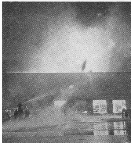
AP Wirephoto GROCERIES GO UP —In what was described as San Francisco's biggest blaze since the fire caused by the 1906 earthquake, this huge Safeway Stores warehouse went up in flames on August 30. Thirty-three firemen were injured while battling the fire. Officials reported the loss at $3,000,000
