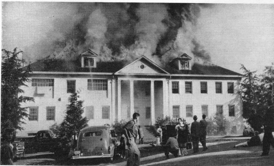
OREGON MENTAL HOSPITAL BURNS — $3,000,000 fire at Salem swept from basement to roof in three minutes on May 18. There was no loss of life because heroic nurses, well-trained for emergencies, led all patients to safety
