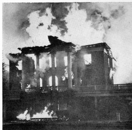
Associated Press AUDITORIUM SILENCED — Flames engulf auditorium and dormitory building of Virginia Teachers College, Farmville, early on the morning of March 6
