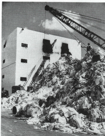
Miami Herald MORNING-AFTER MESS —Fire in a trash box in warehouse of Miami Herald spread to rolls of newsprint and gave local firemen their toughest struggle in years. Paper rolls swelled to half again their normal size, blocking windows and doors and forcing the firemen to cut holes in 15-inch concrete roof
