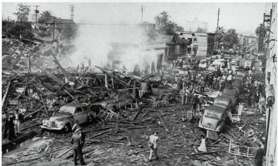
UNPROVED PROCESS CAUSED BLAST —which damaged twelve city blocks when 300 gallons of perchloric acid solution exploded in a Los Angeles electroplating plant. Force was equal to that of one and a half tons of nitroglycerine
