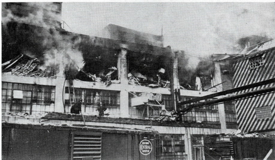
Wide World FIFTEEN PERSONS DIED on September 7 following an explosion of cornstarch used in candy making at the huge Brach Candy Company's plant on Chicago's West Side
