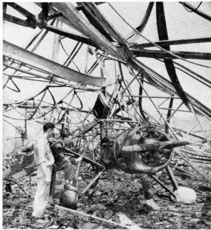
International GROUNDING —Charred engine and landing gear are all that remain of one of fifty airplanes which burned during recent half-million-dollar fire at Teterboro (N. J.) Airport. Twisted steel girders of hanger attest to heat of the blaze
