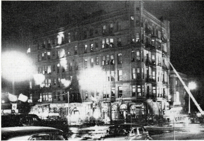
BLAZE BEGAN IN BASEMENT —Forty persons were carried to safety from the Hotel Martin in Milwaukee on February 24. Another 100 left the fifty-nine-year-old brick and stone structure by fire escapes and stairways. There was no panic as trapped guests waited at windows for firemen's help. Many were unconscious from smoke when rescued
