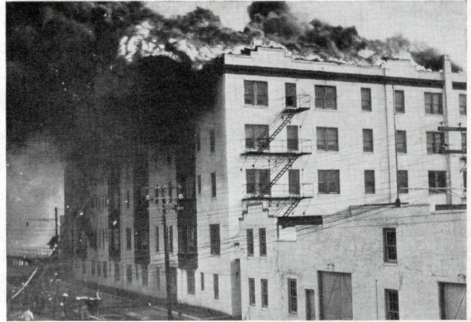
SMOKE STEALS SHOW FROM SURF —Firemen had to work hard and fast to save the Delaware Hotel in Ocean City, N. J., on February 15. Fortunately there were no guests in the 175-room unsprinklered resort hotel when the smoky blaze broke out. A. D. Baggs, manager of the establishment, estimated that damage amounted to about $150,000
