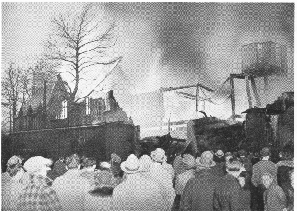
SPRINKLERS SHUT OFF—so this plant burned to the ground, and press reports stated that the firm would go out of business. The sprinkler system was shut off temporarily because of freezing. Protection, to be effective, must be continuous, for fire has a habit of striking when protection defenses are relaxed.
