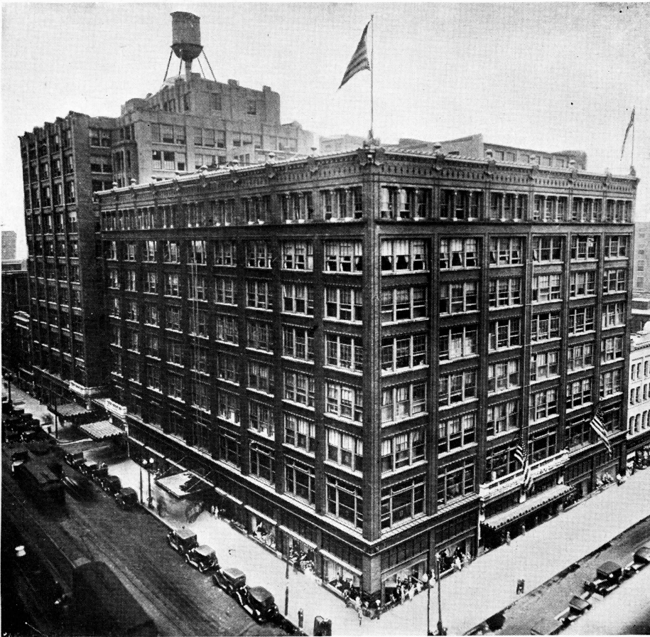
L. S. Ayres Company, the leading department store of Indianapolis, ranks among the most progressive in the United States. The firm has had A. D. T. protection for many years and uses virtually all forms of service. These include Night Watchman Supervision and Manual Fire Alarm service, including the Watchman's Telephone feature, Sprinkler Supervisory Service, Aero Automatic Fire Alarm, Burglar Alarm and Police Call.
