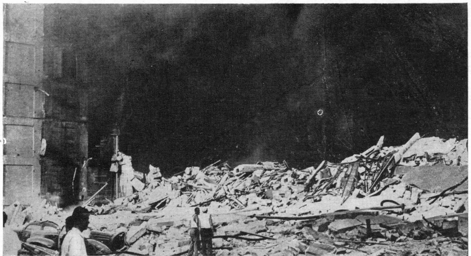
International FATAL BLAST —This pile of debris is all that remained of a six-story building at Kearney, N. J., after explosion caused by a spark igniting volatile vapors
