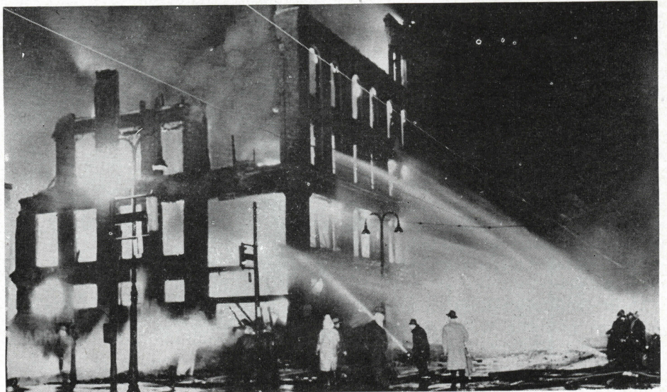
TOLEDO HAS BIG FIRE—This $500,000.00 blaze—the second in the city in two weeks—gutted several downtown stores and threatened the business section
