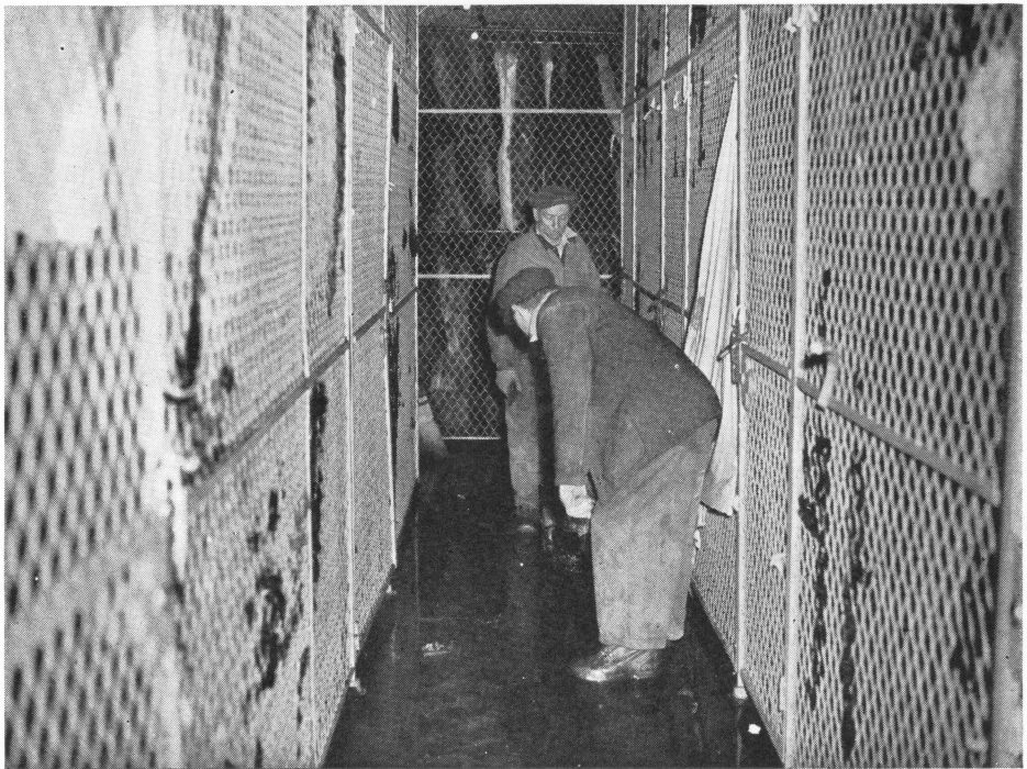
MOPPING UP—Employees of the warehouse mop up water discharged by the sprinkler system which, though it wet some of the garments, did an effective job of holding the fire in check until the firemen arrived. The vault was divided into about fifty compartments of varying size similar to the one in the picture.
