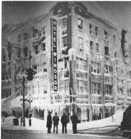
Pictorial COSTLY HOTEL FIRE —The Hotel Windsor in Poughkeepsie was gutted by a fire on February 18 while water from hoses froze in the sub-zero weather
