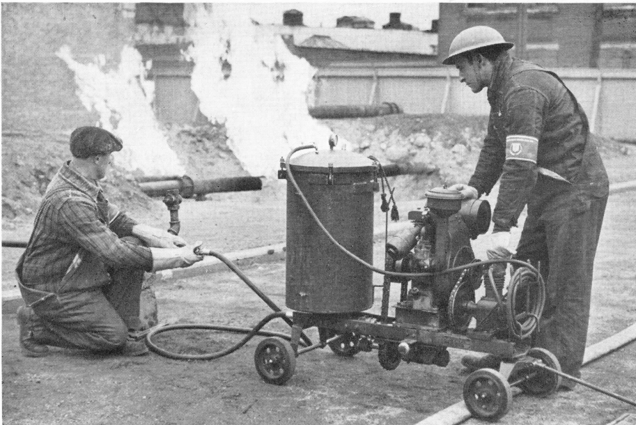
GETTING READY FOR AIR RAIDS—In preparation for the gas leaks and fires that occur after bombings the Brooklyn Union Gas Company is training more than 2,000 volunteers. Here two emergency trainees operate a machine which shoots heavy grease into broken main and shuts off gas, stopping the fire
