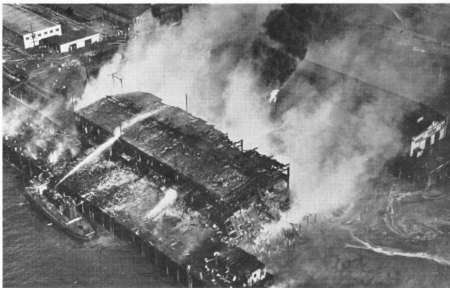
FIRE DESTROYS SEATTLE PIER—Aerial view of the recent $170,000 fire at the Connecticut Street Terminal Pier, Seattle, Wash. Eighteen fire companies and four fireboats fought the blaze but were unable to check the flames
