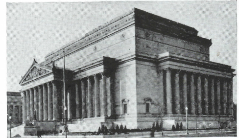
ARCHIVES BUILDING "Aero" Automatic Fire Alarm, Burglar Alarm, Watchman Supervision, Manual Fire Alarm
