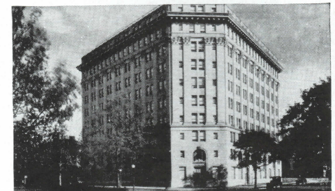
HOME OWNERS LOAN CORP. BLDG. "Aero" Automatic Fire Alarm, Burglar Alarm, Watchman Supervision, Manual Fire Alarm
