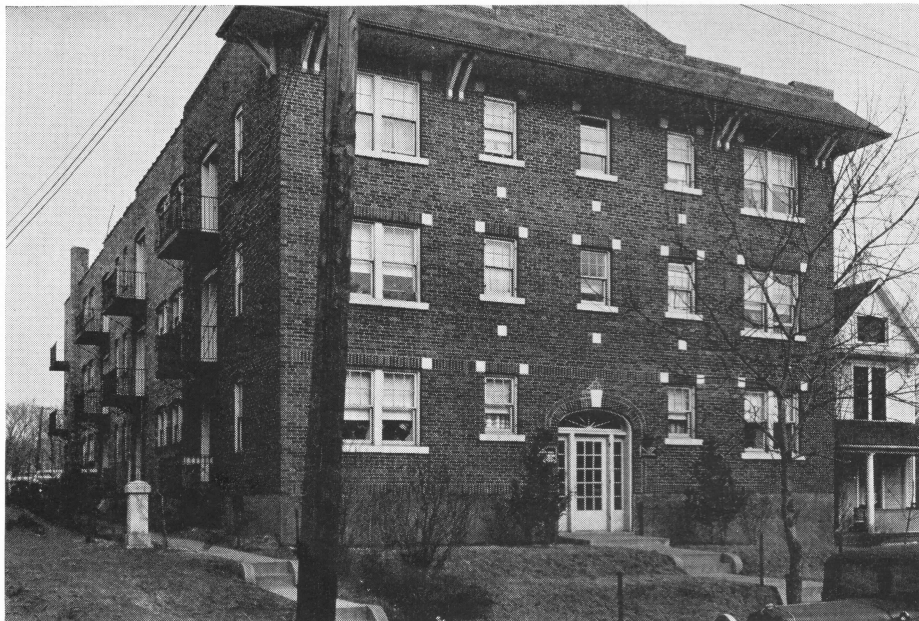
NO WORRIES ABOUT FIRE need beset either the tenants or the owners of this modern apartment building recently opened in Maplewood, Mo. The basement, public halls, and similar hazardous areas throughout the building are protected by an Aero Automatic Fire Alarm System
