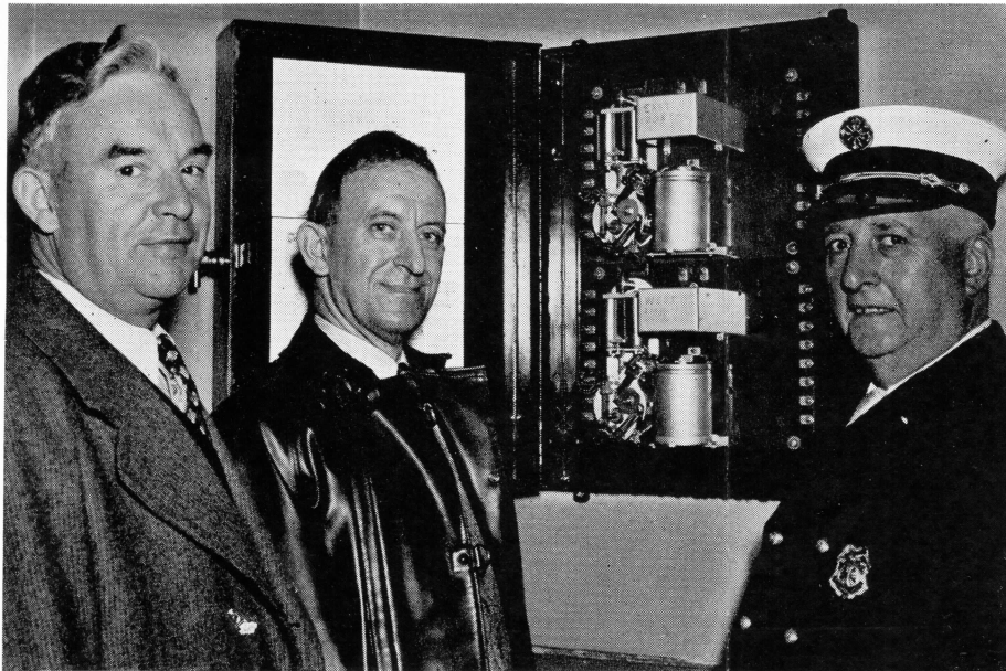
AERO PROTECTS CINCINNATI MUSIC HALL—Local officials pose before alarm transmitter after demonstration of the recently installed Aero System. Left to right: Assistant Fire Chief Chris Williams, Deputy Building Inspector Albert Frazer, Salvage Corps Superintendent E. J. Ader
