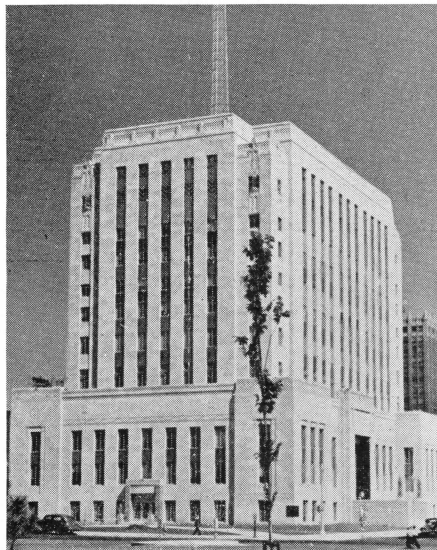
OKLAHOMA COUNTY BUILDING, Oklahoma City, where jail section, one of most modern in the country, recently was equipped by A.D.T. for reporting by guards
